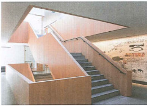
7 Holz prägt die Innenräume. | The interior is characterised by wood.
